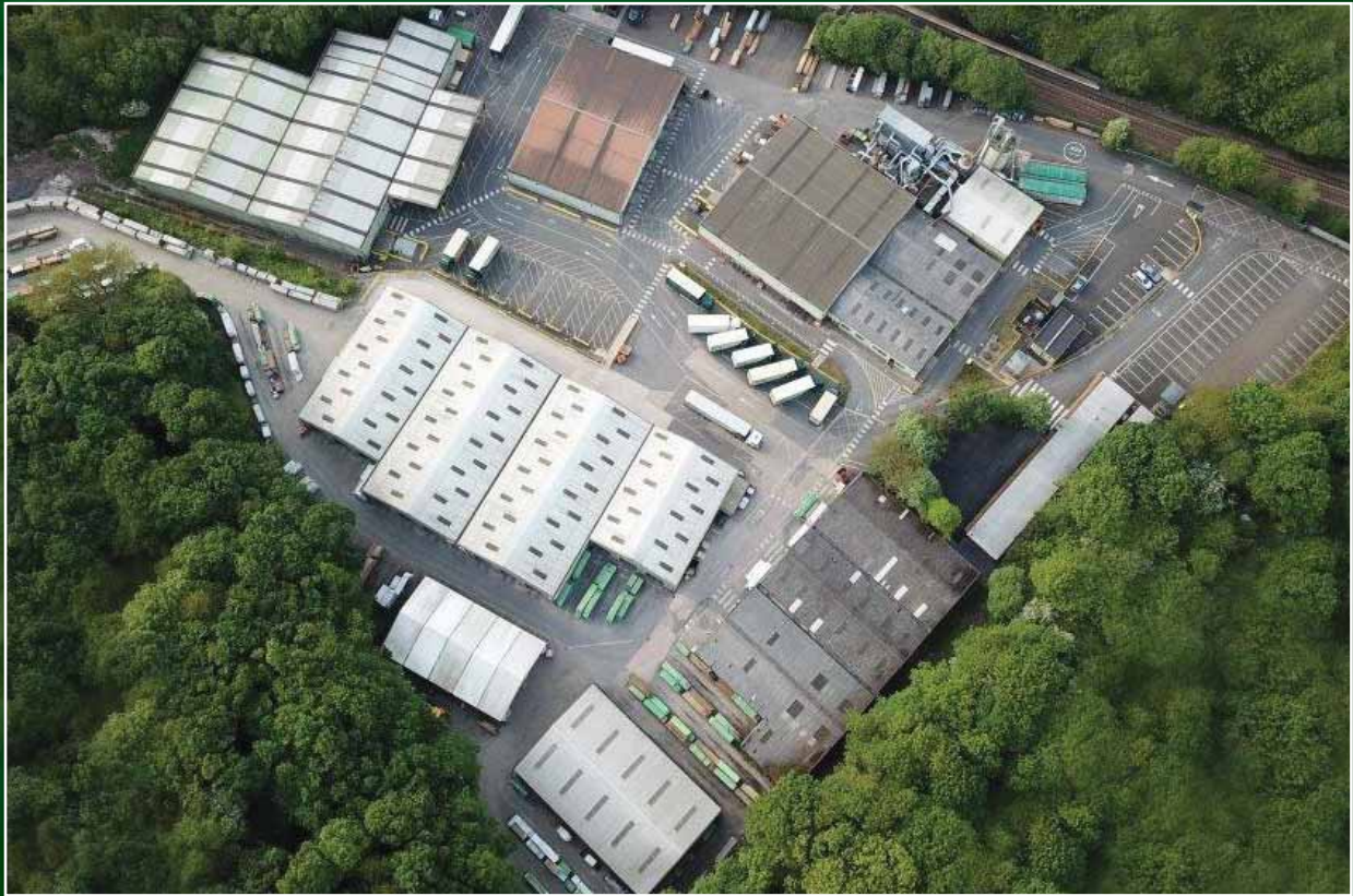
Palmer Timber Head Office and 13 Acre Site
